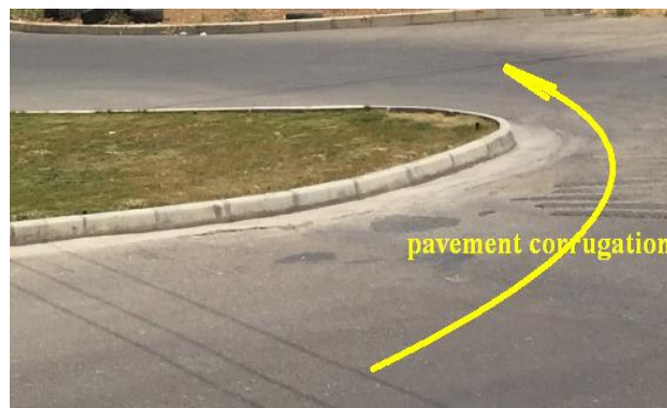
Figure (9) Pavement corrugation around the divisional island
