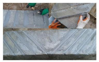
Figure (3) Groove Cutting Process
