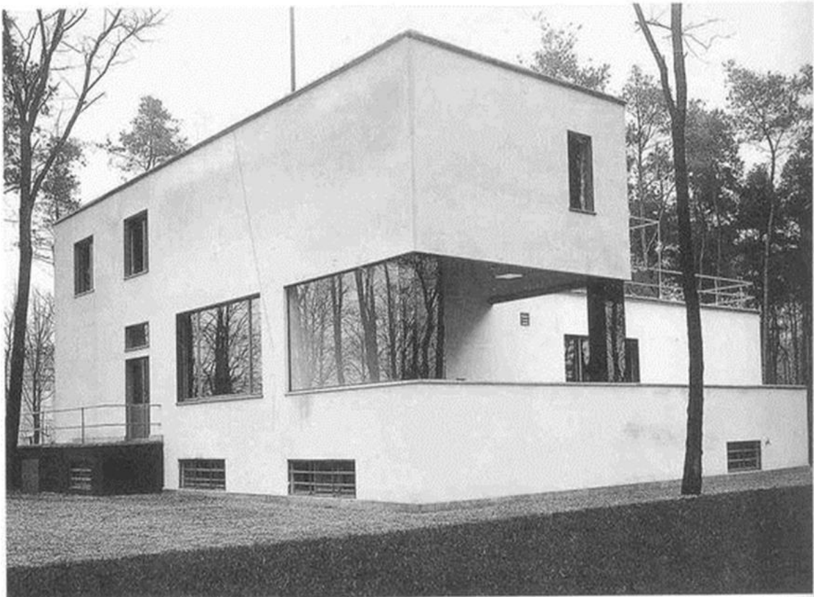
Figure 7: The 1st master house, for Walter Gropius showing black glass cladding over column before WWII, Source: ( http://www.uncubemagazine.com/blog/13113621 )
