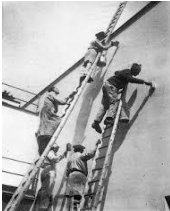
Figure 13: Lime plastering by Hens Meyer's students when he was second director of the Bauhaus from 1928 to 1930. Source: Pinterest ( https://www.pinterest.de/pin/171770173261239931/?lp=true )
