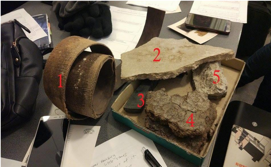
Figure 6: Materials found in Bauhaus Dessau museum building, 1. Triolin, 2. Magnesial flooring, 3. Black opaque glass cladding, 4. Torfoleum and 5. Concrete. Source: Sayed Ahmed during survey in 2016
