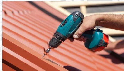
Fig. 7 Use of an impact Driver to tighten the Bolt in
