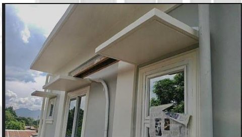
Fig. 3 the reinforced concrete awning
